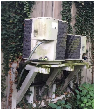
(north elevation prior to repair)
