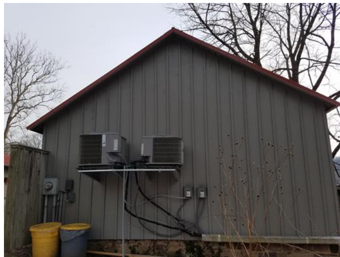
(north elevation of Commission office after repairs)
