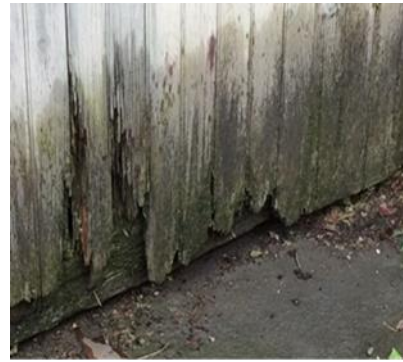
(exterior water damage)
